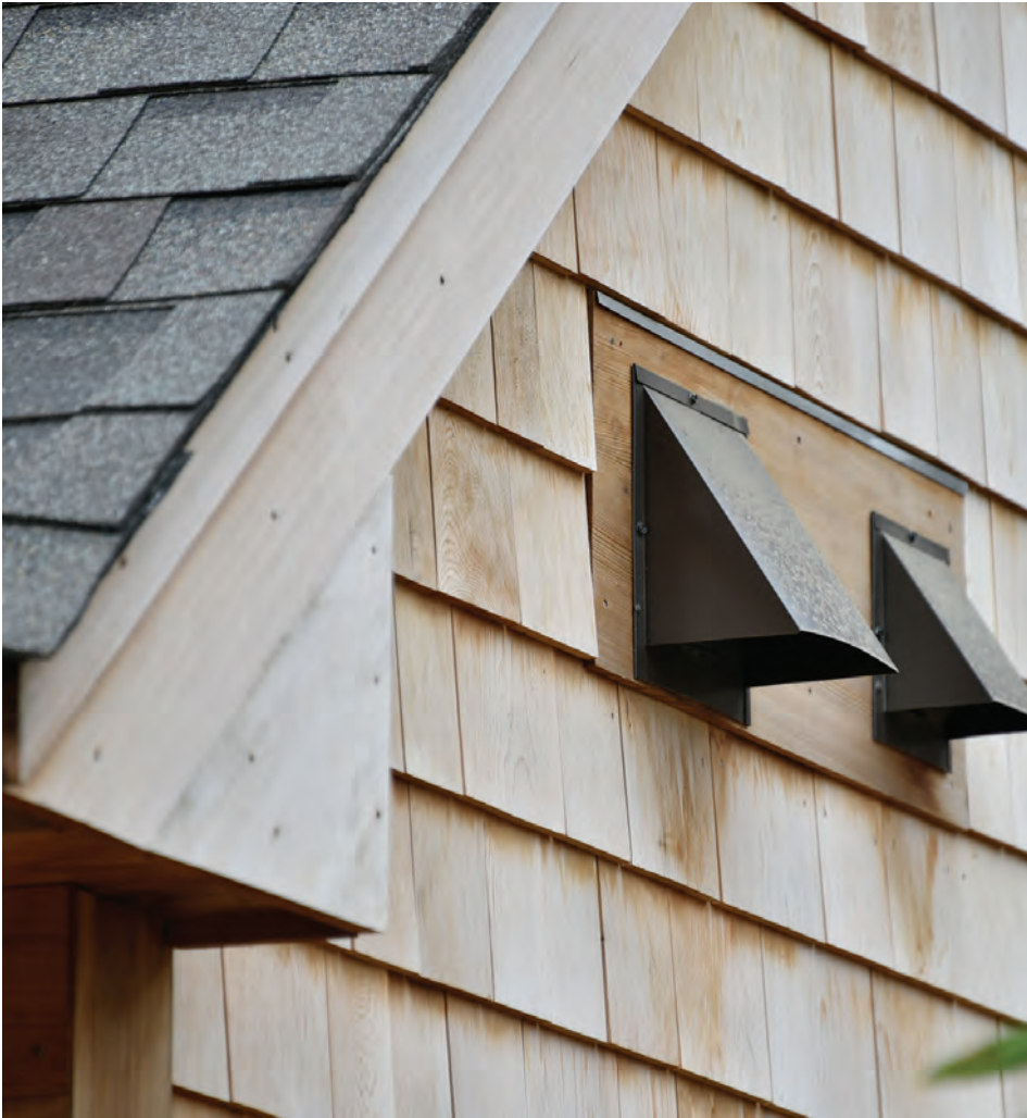
CLOCKWISE, TOP TO BOTTOM: Cedar trim costs a little more up front, but in the lifetime of the building it will cost less because it won't have to be painted. Brackets are fir and the decking is sustainably harvested mahogany from Malaysia, which, Derrill notes, has a well-established and long-term sustainable forestry program. Side-by-side exhaust vents – one for the air system, one for the clothes dryer.
