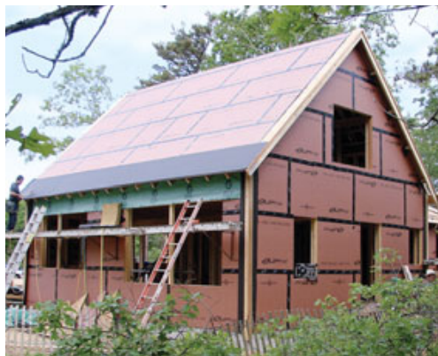
Figure 8. Taped Zip System sheathing — applied continuously on the walls, over the plumb-cut rafter ends, and up the slope of the roof — provides the primary air barrier. Note the layer of housewrap under the eaves (left), installed in advance as the rafter tails were being added. Later, the entire shell was covered with housewrap.
