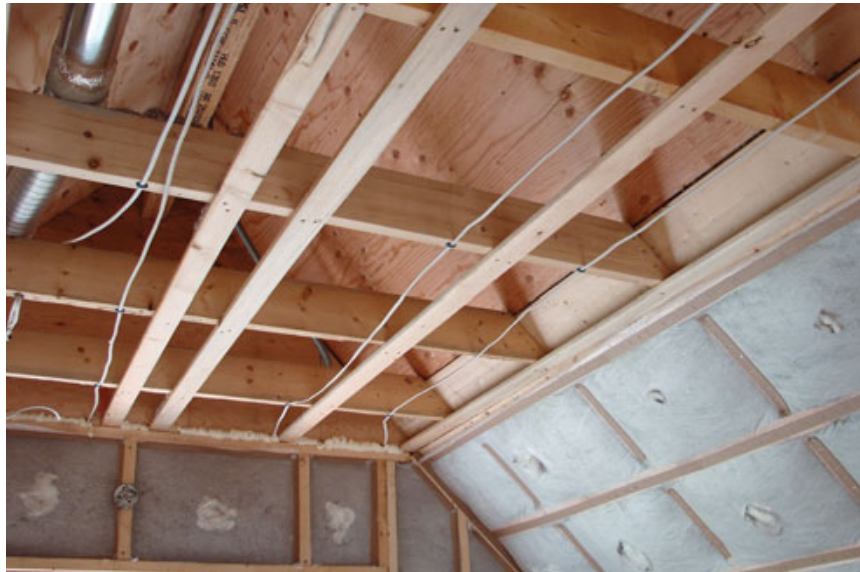
Figure 10. Unused attic spaces are part of the home's conditioned space, so the rafters are insulated up to the ridge. Note that plywood is used in the attic to hold the insulation in place where there is no drywall.
