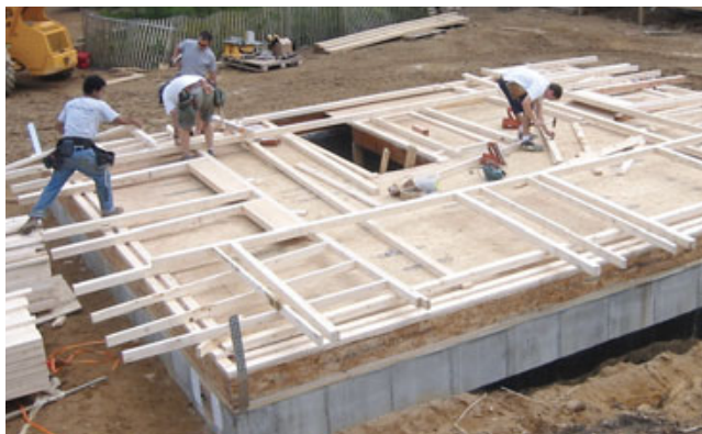
Figure 5. Precut studs, joists, and rafters saved labor and substantially reduced waste. Even the rafter plumb cuts were made by the lumberyard.
