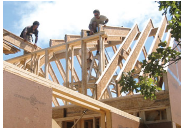
Figure 4. Double 2x4 walls (left) and 14-inch-deep wood I-joint rafters minimize thermal bridging through the frame. Note that the rafters' bottom plumb cuts are flush with the walls (above).
