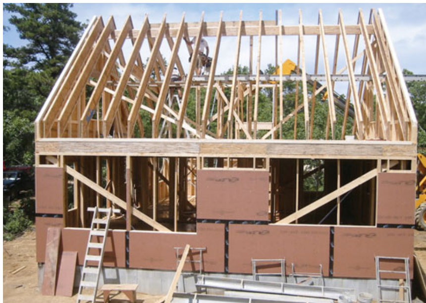
Figure 8. Taped Zip System sheathing — applied continuously on the walls, over the plumb-cut rafter ends, and up the slope of the roof — provides the primary air barrier. Note the layer of housewrap under the eaves (left), installed in advance as the rafter tails were being added. Later, the entire shell was covered with housewrap.
