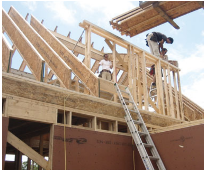
Figure 4. Double 2x4 walls (left) and 14-inch-deep wood I-joint rafters minimize thermal bridging through the frame. Note that the rafters' bottom plumb cuts are flush with the walls (above).
