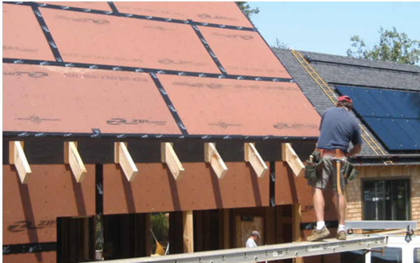
Figure 9. To avoid the gaps in the air barrier that typically occur where the rafters cross the top plates, the author decided to apply false rafter tails to the outside of the airtight shell (top), first installing a course of a self-adhering flashing membrane to seal fastener penetrations. Cypress backers were screwed to the back of each tail, then the assemblies were screwed through the sheathing into the rim joist. A TimberLok screw driven diagonally through the top of each tail into the rim helps resist downward forces. Pine-board sheathing completes the open-tail look.
