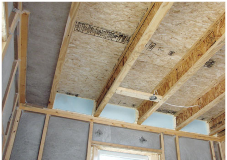
Figure 7. The second-floor band joists required blocks of 1-inch polystyrene, spray-foamed in place, to meet insulation goals.
