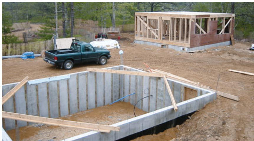
Figure 2. Wedged-shaped battens made of pressure-treated lumber were fastened to the inside of the foundation forms 2 feet on-center. A double layer of 1½-inch polyisocyanurate foam board is attached to the battens with screws and plastic washers.
