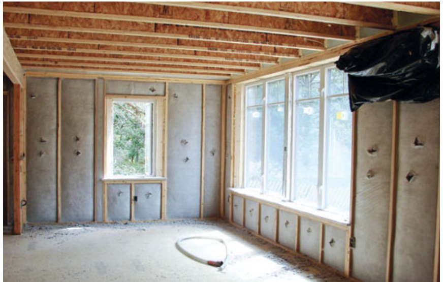
Figure 6. Because of the 9½-inch cavity created by the double 2x4 walls, the blown cellulose achieves an R-value of 31. The sides of the deep window wells are beveled 45 degrees to ensure that they let in plenty of light.
