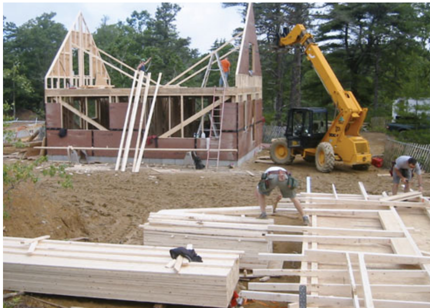
Figure 5. Precut studs, joists, and rafters saved labor and substantially reduced waste. Even the rafter plumb cuts were made by the lumberyard.
